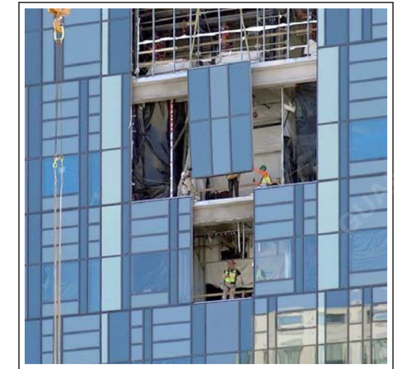
Unitized curtain wall lifting
