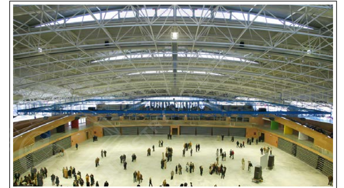
Grid space steel structure systems
