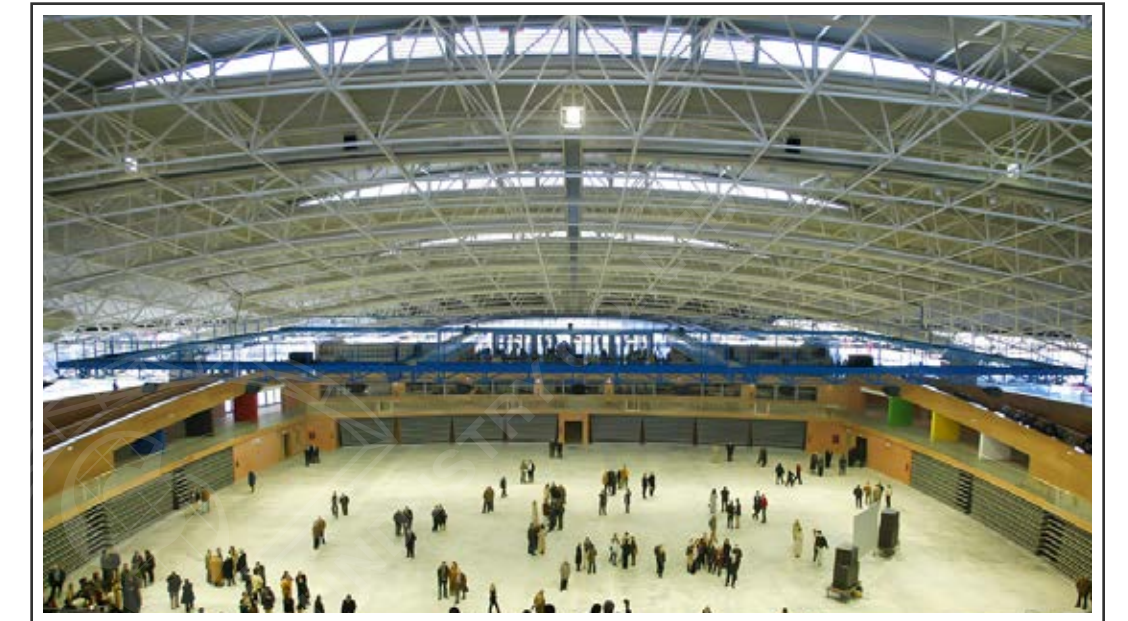
Grid space steel structure systems
